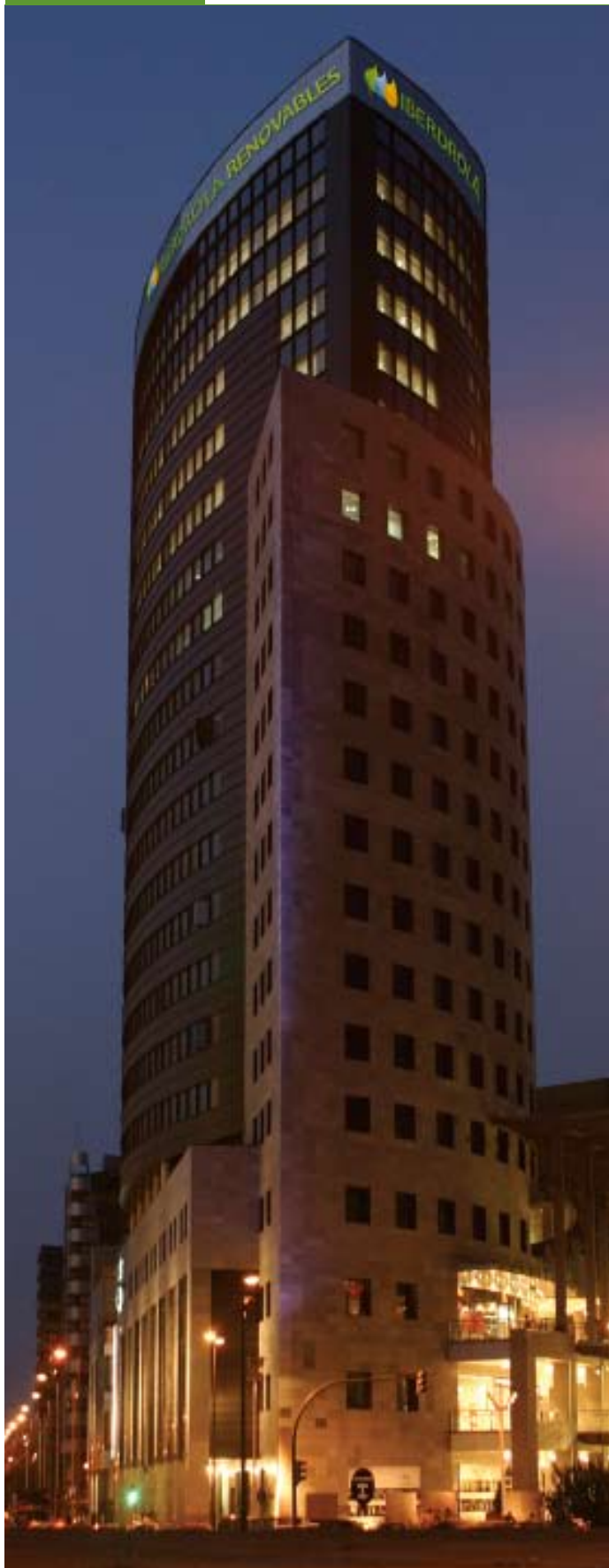
IBERDROLA RENOVABLES headquarters (Valencia).
