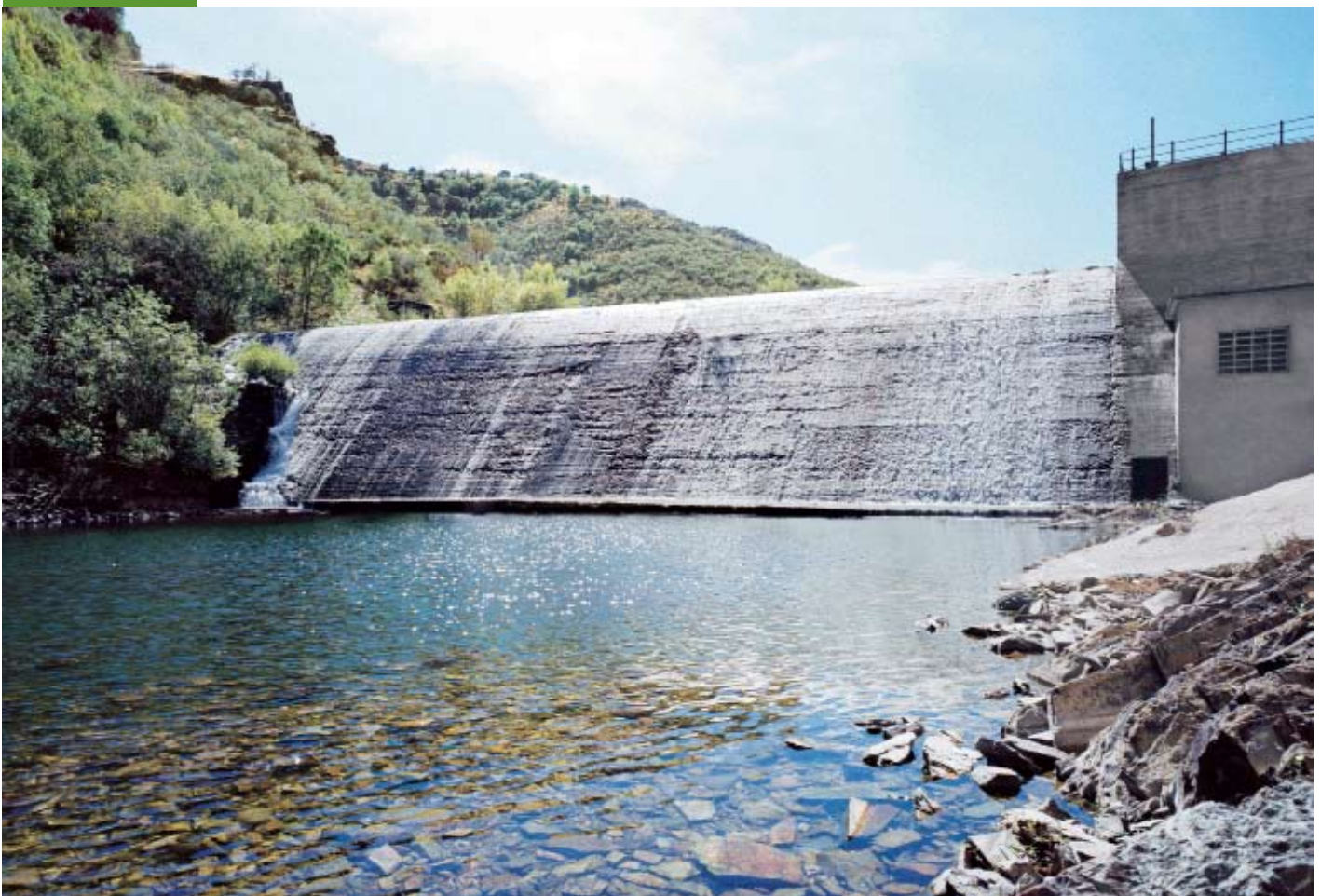
La Retorna mini-hydro plant (Logroño).
