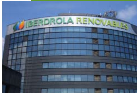
Iberdrola Renovables headquarters (Valencia)
