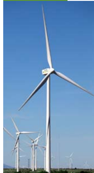
Maranchón wind farm in Guadalajara (Spain).
